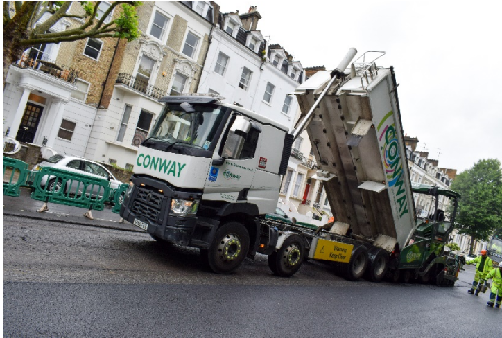
Westminster, Sutherland Avenue 80 percent recycled asphalt trial
