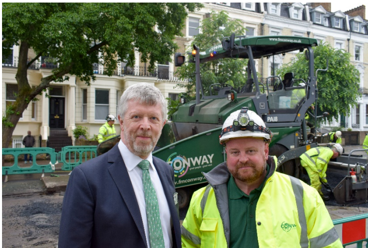
Westminster City Council Cabinet Member for City Management and Highways, Tim Mitchell & FM Conway Technical Manager, Mark Flint
